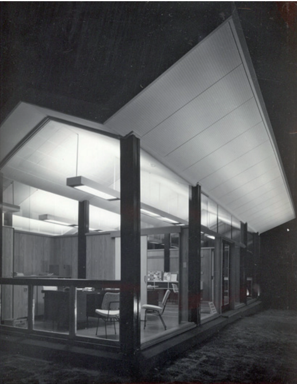
Above and Left: The transparency of the building as a "jewel box" is obvious without the impeding view of diagonal bracing. The glass, where possible, was butt jointed to maintain complete transparency to the interior. The florescent light fittings were also especially designed as timber boxes to "throw" light upwards as well as down through diffusing grids. Since the company was also an agent for plywoods, it was decided to use waterproof acoustic ply on the underside of the front "awning" splay of the roof in order to reduce reflections of noise into the building from the busy road nearby.
